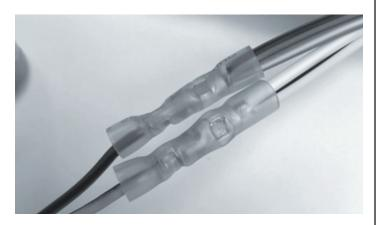
The butt connectors are heat shrink style – so using a torch or hot air gun, shrink the connectors.
